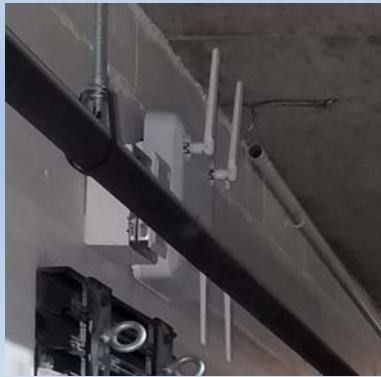
Access Points mounted to wall and use directional antenna.
